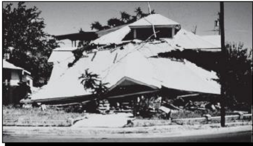
Additional damage from aftershocks
