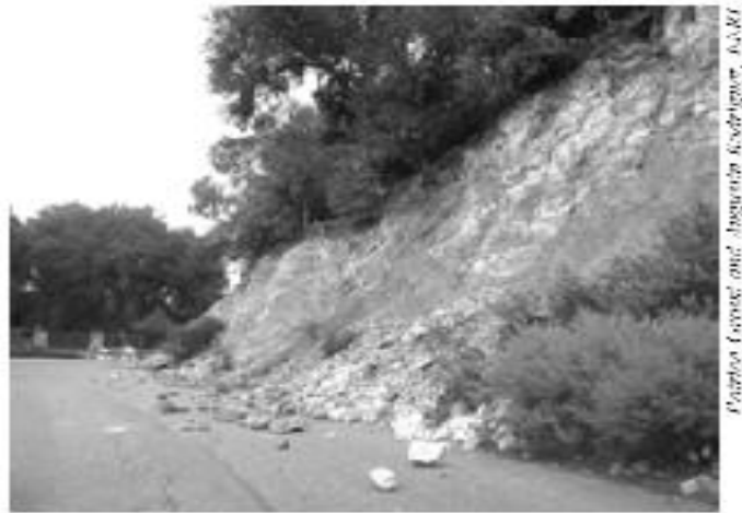
Figure 37 - Landslide. San Simeon Earthquake, December 22, 2003 Landslides on San Gregorio Road in Atascadero, California, only a short distance away from where the homes with the most damage were located.
