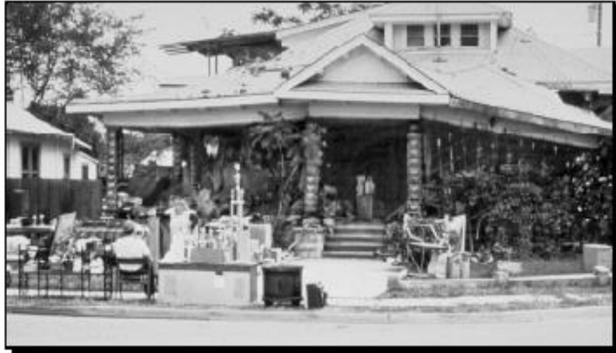
Damage from magnitude 6.7 earthquake
