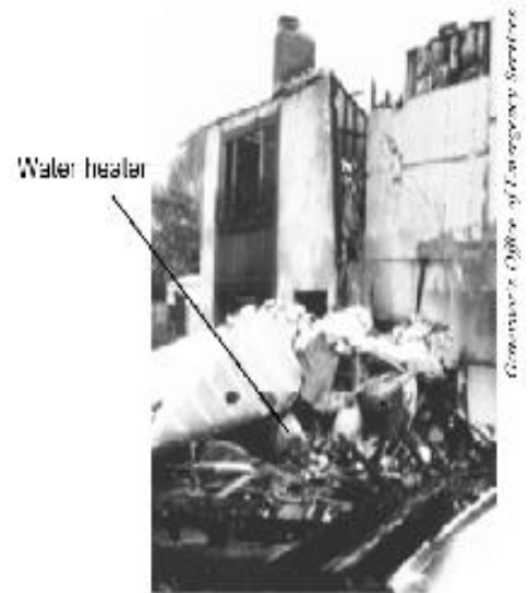
Figure 10 - The unbraced water heater in this home fell during an earthquake; the resulting fire destroyed the home.
