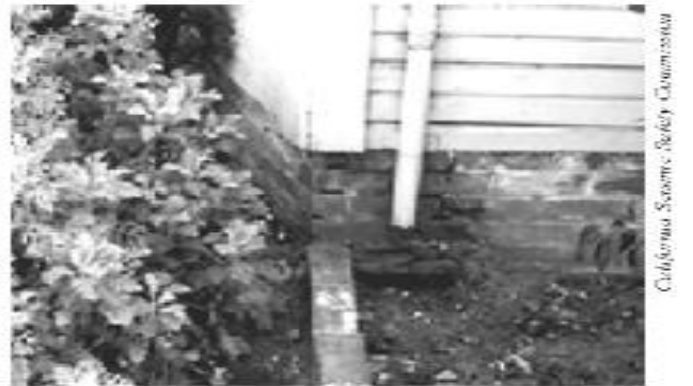
Figure 20 - Note the bricks exposed in this unreinforced masonry foundation.
